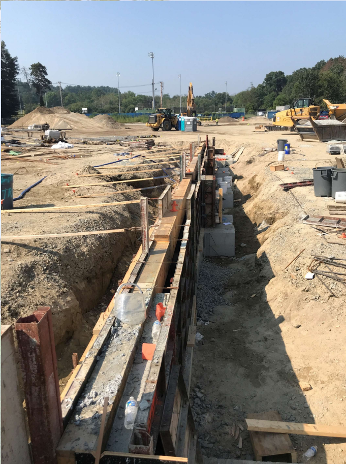
Area B Formwork
