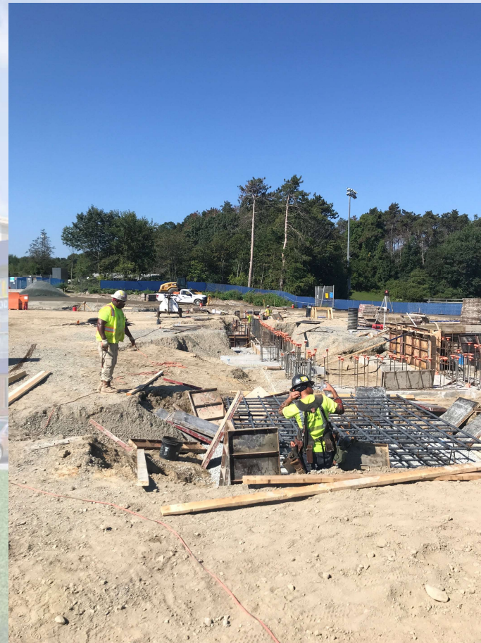
Area B Rebar / Placement
