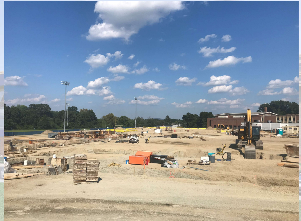
General site overview
