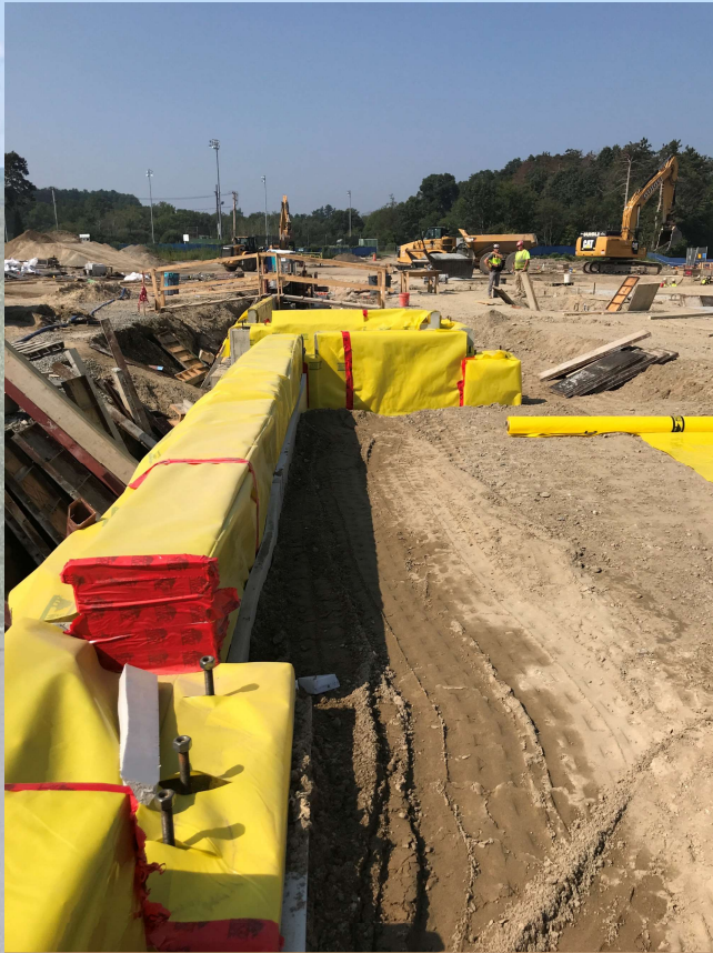
Area C Vapor Barrier
