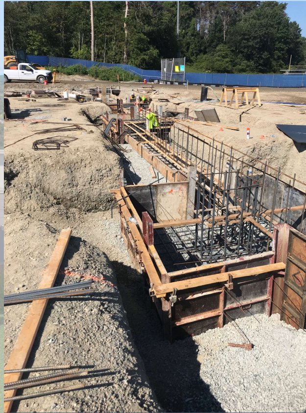
Formwork Area B
