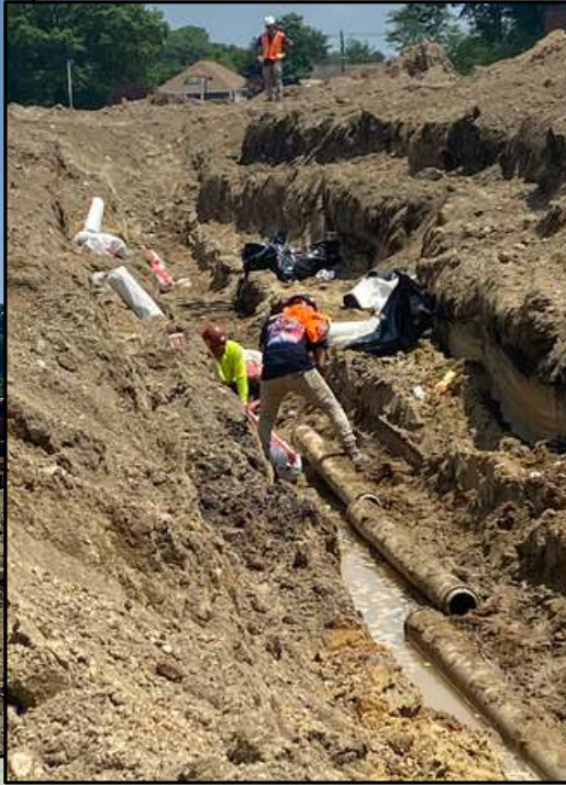
Removal of UG Transite Pipe
