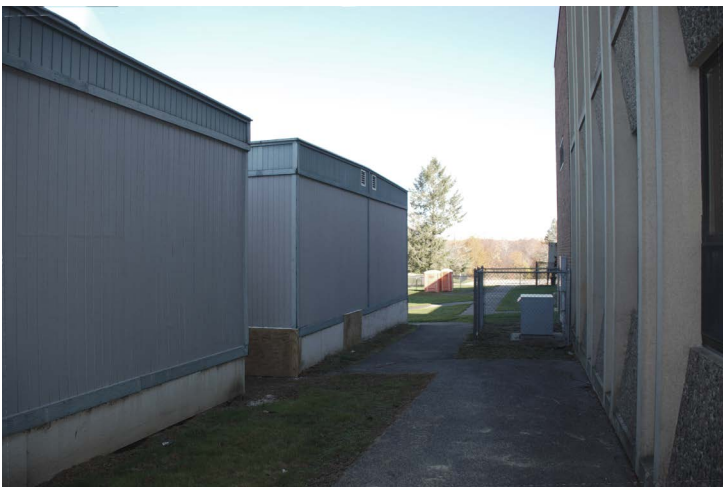
Modular classrooms have become permanent fixtures, despite signs of deterioration
