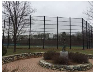
Photo 10: Patio and Baseball Fence
