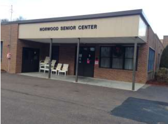
Photo 2: Front Entrance to Norwood Senior Center
