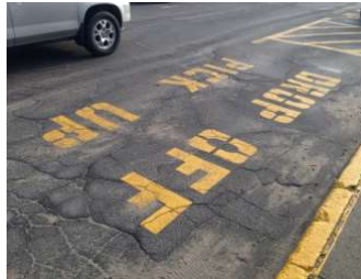
Photo 5: Drop Off Area
