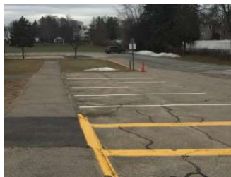
Photo 5: Northwest Parking Lot
