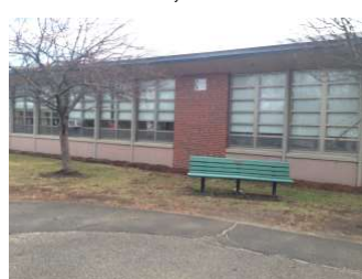
Photo 20: Trees Along West Side of Building
