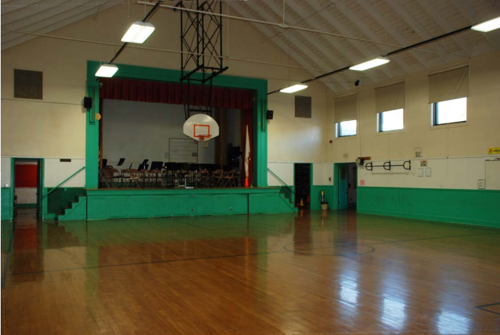
The roofing system over the gymnasium is pitched and covered with asphalt shingles
