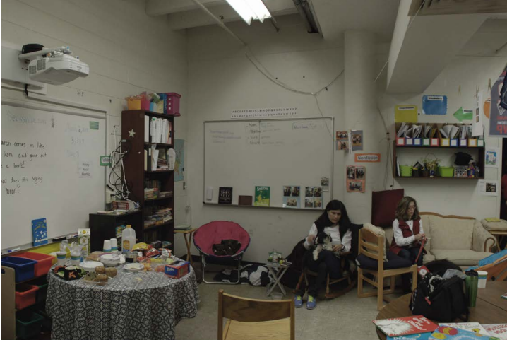
Rooms originally unintended as classroom space are being used as such, without access to fresh air or daylight
