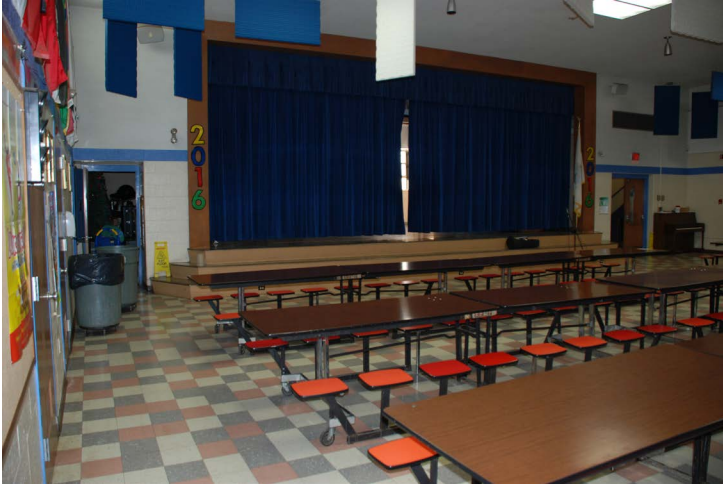
Student dining is one such area still containing Vinyl Asbestos Tile (VAT), a hazardous material
