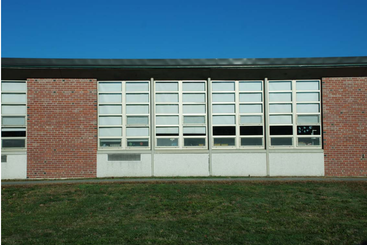
The exterior envelope is composed of brick bays and continuous stacked window units within a pre-cast concrete infill system
