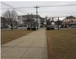
Photo 2: Front Concrete Walk
