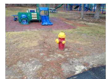
Photo 11: Southwest Fire Hydrant
