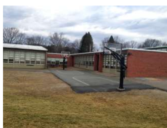
Photo 17: Southeast Basketball Court
