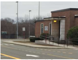
Photo 3: North Accessible Entrance
